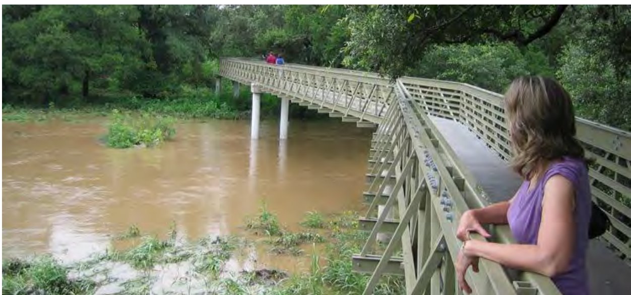
Figure 12. Example of a footbridge in floodway/floodplain
