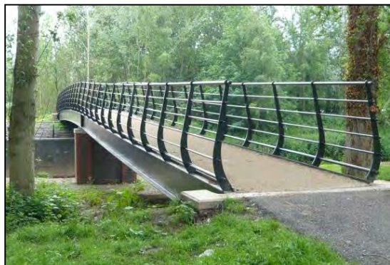
Figure 11. Example of a Beam Bridge
