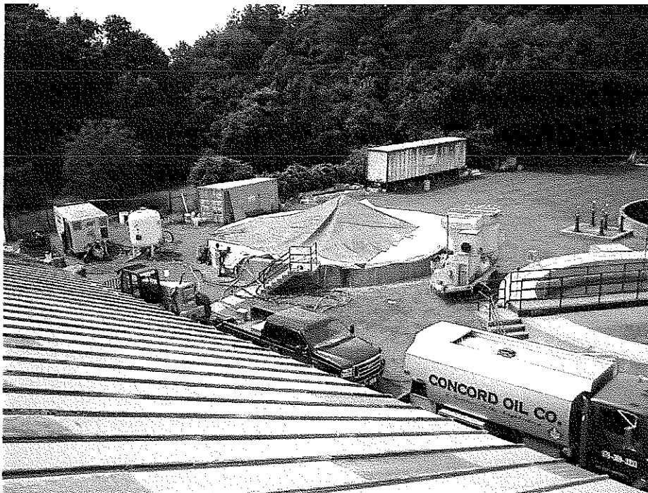
An overview of the # primary clari-thickener undergoing sandblasting in late July.
