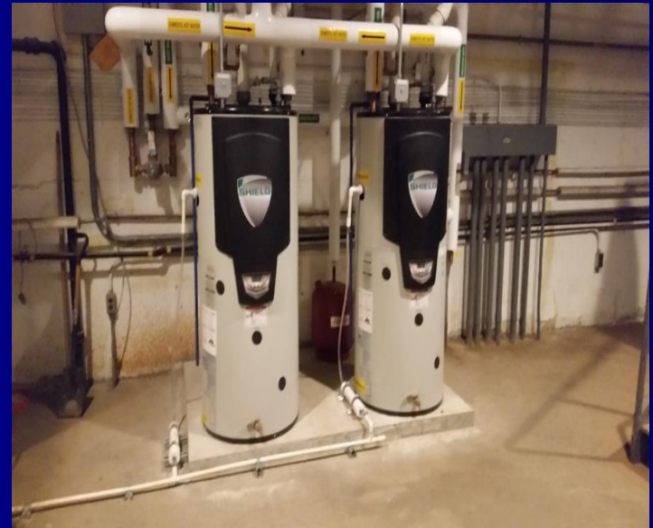
New Lochnivar Condensing Boilers & High Efficiency Hot Water Heaters
