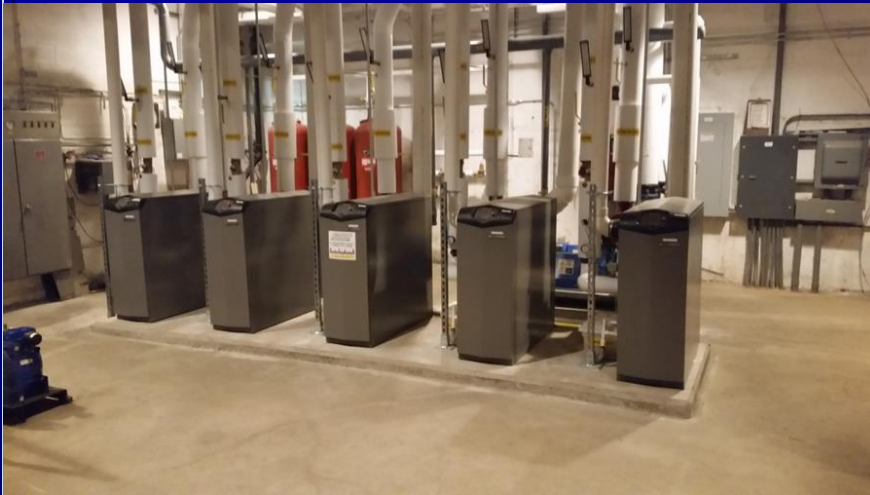
New Lochnivar Condensing Boilers & High Efficiency Hot Water Heaters
