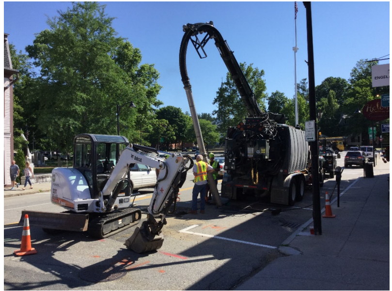
Sewer Service Repair – Main Street
