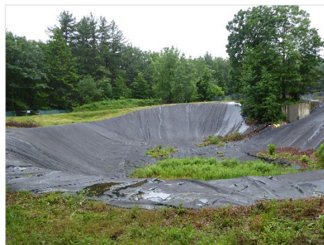
Photo 5: Holding basin area.
