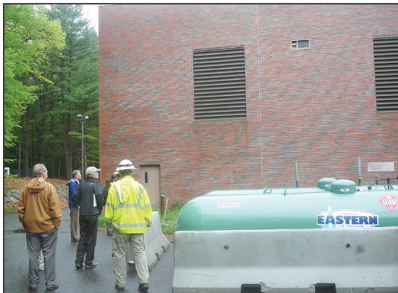
*Fred Seward and engineers view barriers around new natural gas tanks that supply powerful blowers to heat the buildings at 2229 Main St. during the building disassembly. The buildings must be heated to keep fire suppression systems working and to keep snow from collecting on the roof during the winter.*
