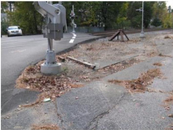
Conant Street crossing looking south.
