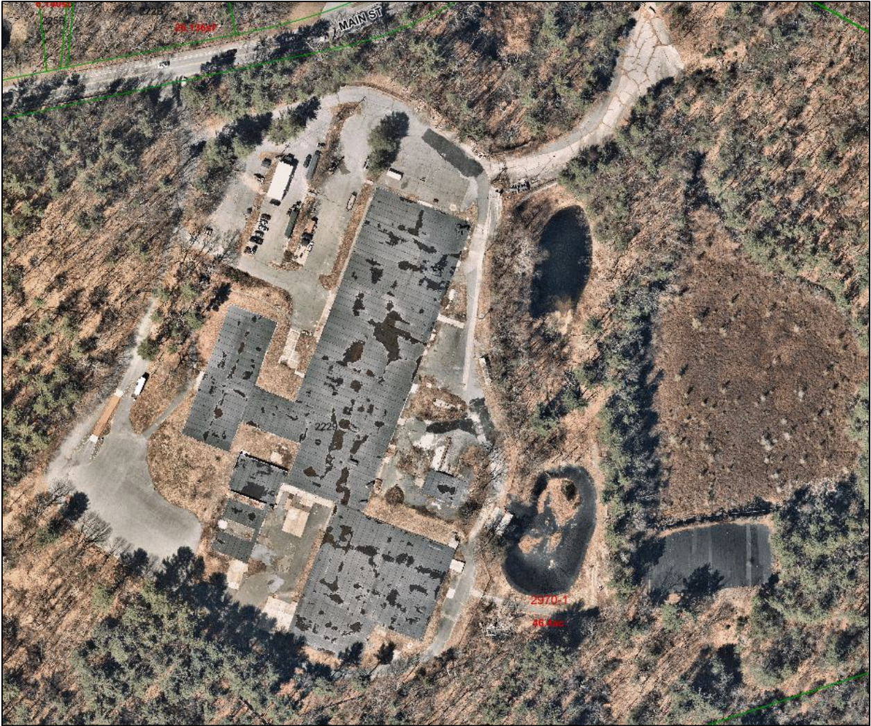
FIGURE 1.3 BUILDING SLABS ADJACENT TO HOLDING BASIN, COOLING WATER RECHARGE POND AND SPHAGNUM BOG
