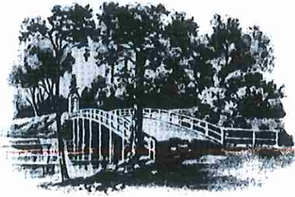
OLD NORTH BRIDGE
