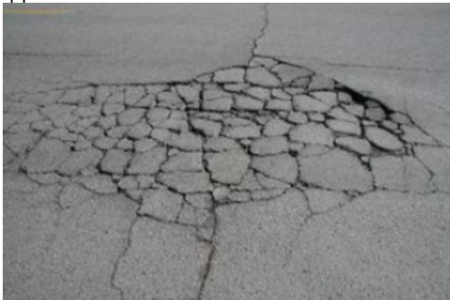
Alligator Cracking:
