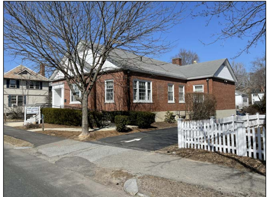
EXISTING - FROM SOUTHEAST
