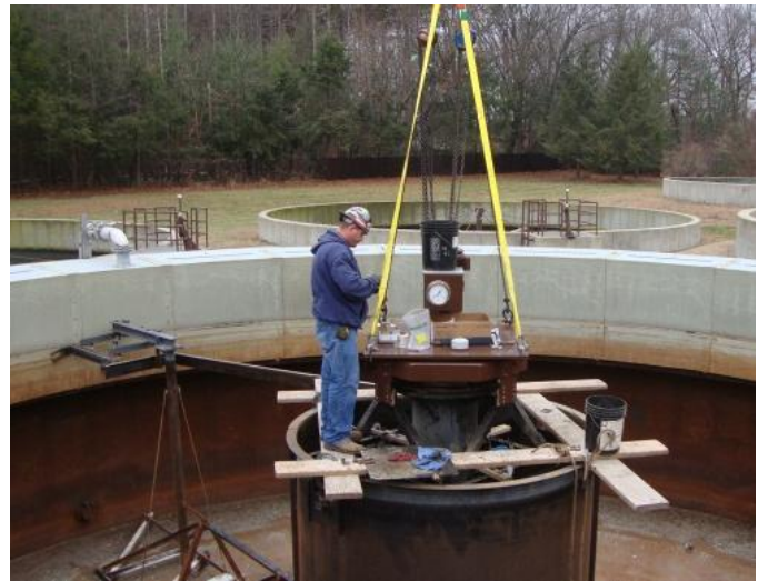
Primary Clari-thickener - Drive Replacement
