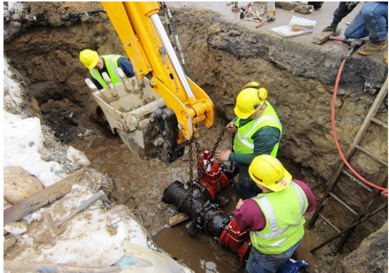
Water Main Valve Replacement
