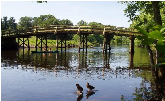
Old North Bridge (Wikipedia)
