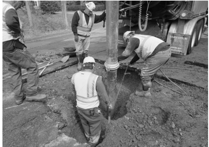
Water Main Repair on Cambridge Turnpike
